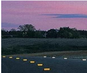
Reflective pavement markers to increase visibility
