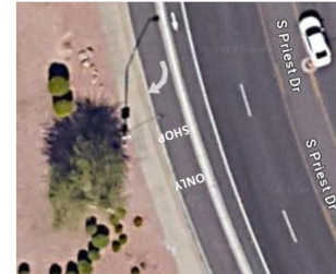
Additional pavement markings in the turn lane leading to shops
