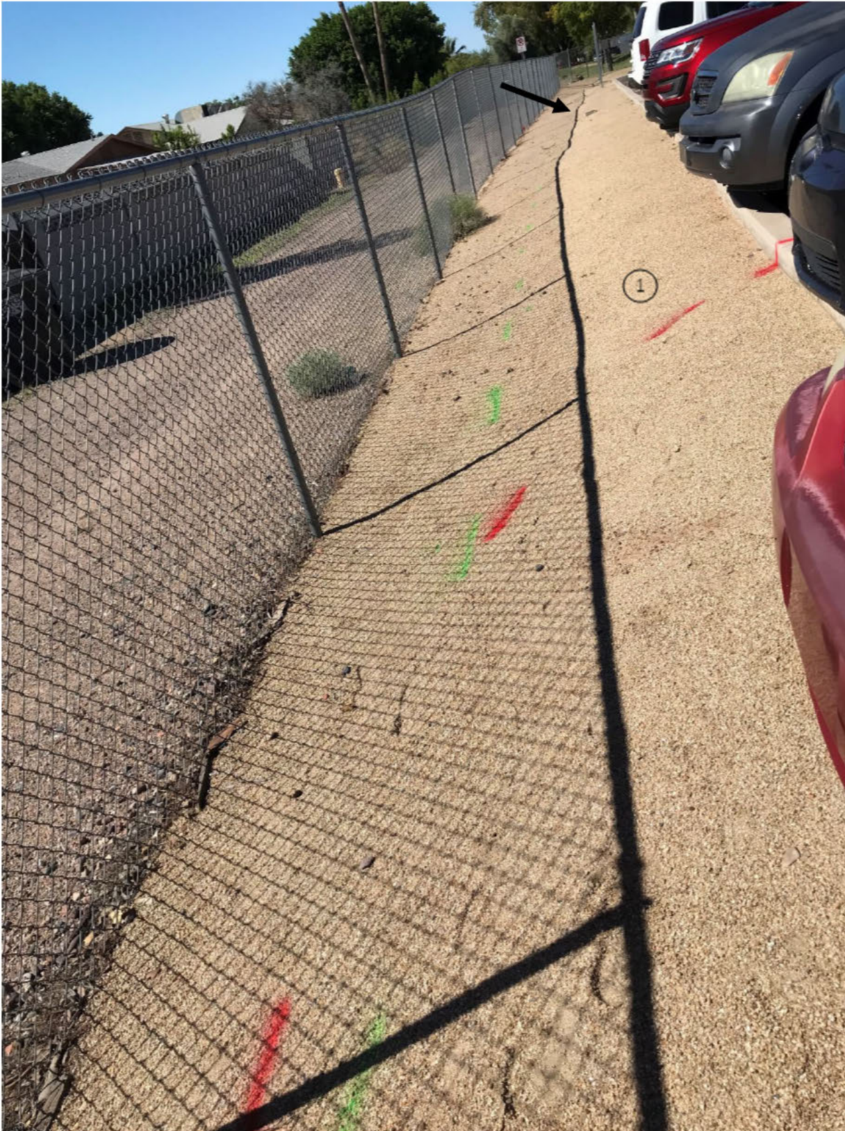
Figure 6. Private Locator Marks from Fall 2018 (Note: Black Arrow is same location as following picture; no lines found in areas 2 & 3)
