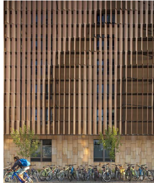
Vertical Fin Shading structure at Tooker Hall, ASU
