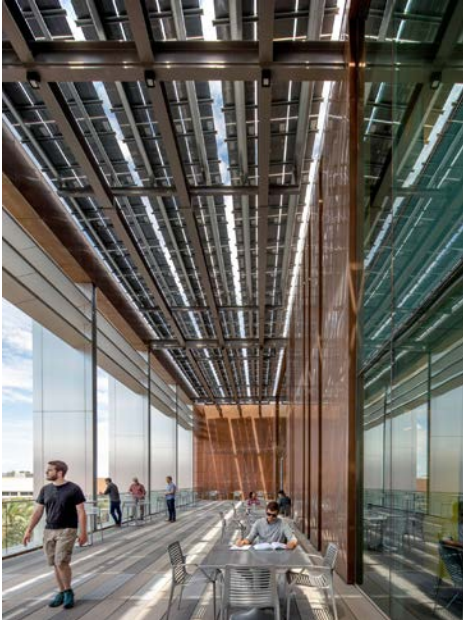
Shading Structure on South Facade at ASU Student Pavilion
