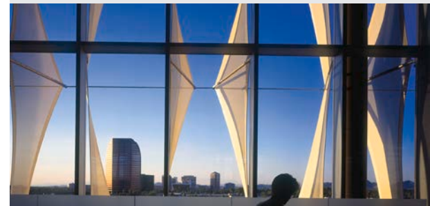
Phoenix central library glazing on North Facade.
