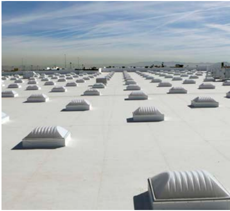
Reflective Roof on a Walmart store, Las Vegas, NV
