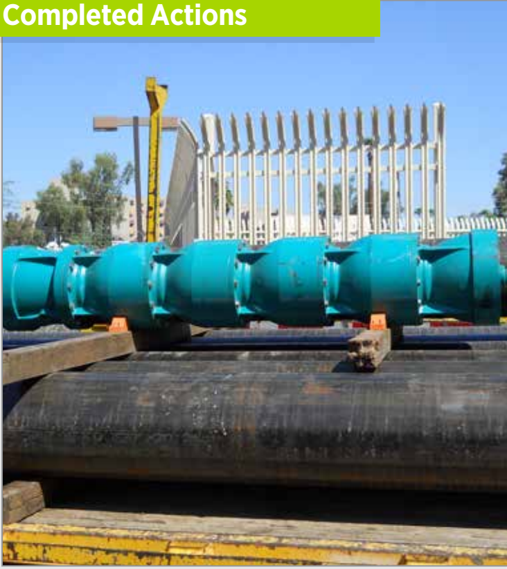
Municipal Utilities water well
