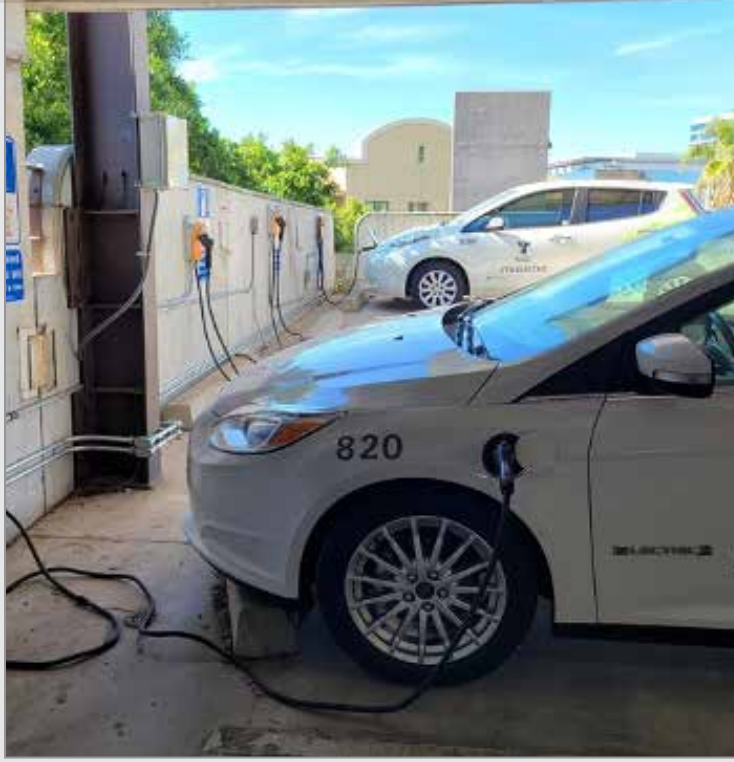
Downtown Police Courts Parking Garage
