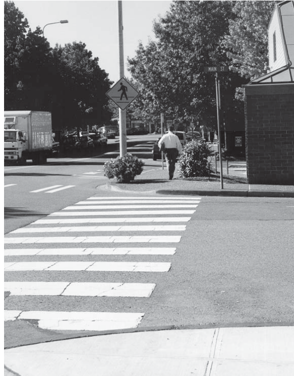
Example of ladder bar crosswalk
