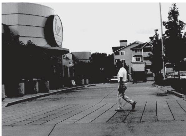
Pavement texture or scoring can be used to delineate the pedestrian travel area in a parking lot.
