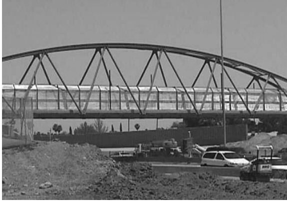
College Avenue Bicycle/Pedestrian bridge
