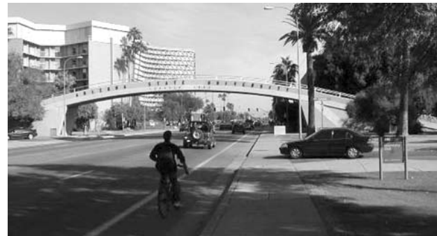
ASU pedestrian bridge.
