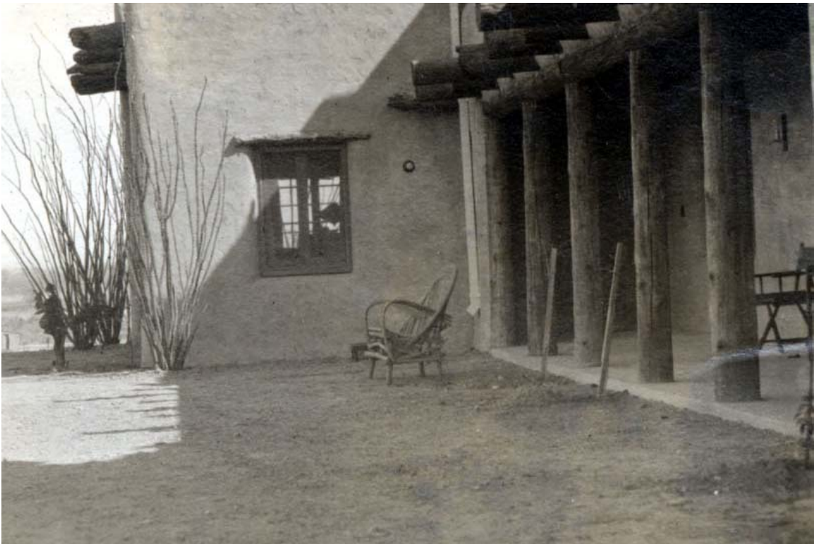
Entry Loggia looking east c. 1931
