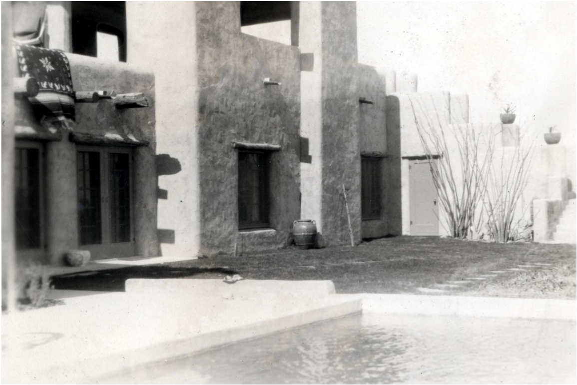
East Terrace looking northwest c. 1931
