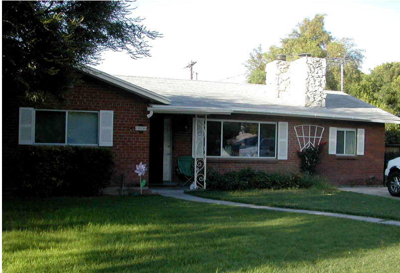
Compatible Carport Enclosure into Habitable Space with openings in scale and proportion, as well as compatible materials consistent with those of the street façade (Site 118)
