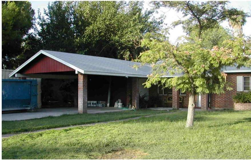
Carport Extension with consistent roof form and material palette (Site 184)
