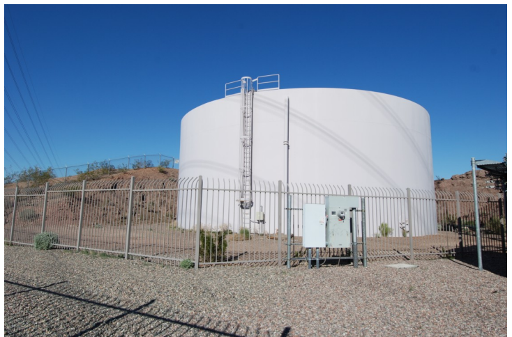
Elevated water storage reservoir
