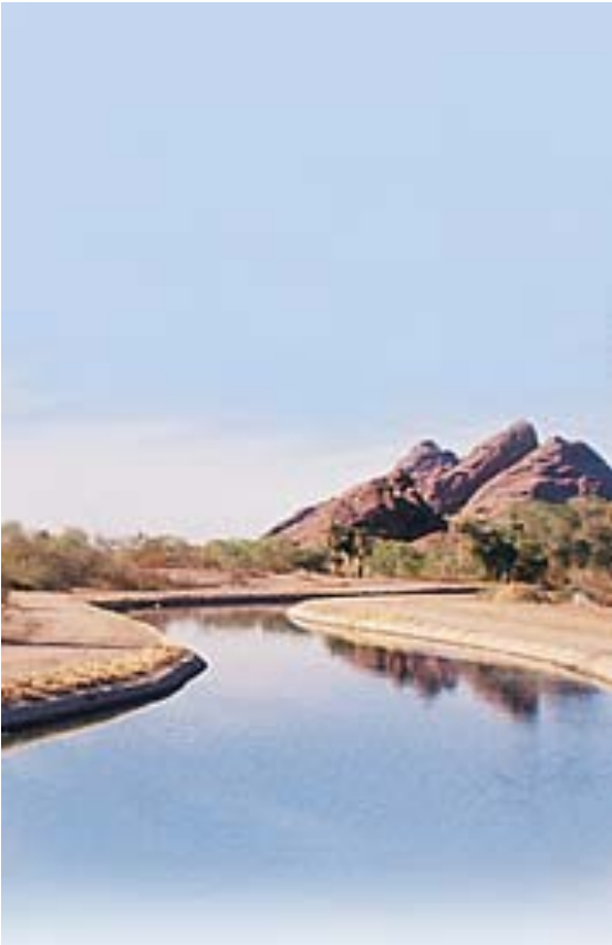
The SRP Cross-cut Canal delivers water to the Martinez WTP
