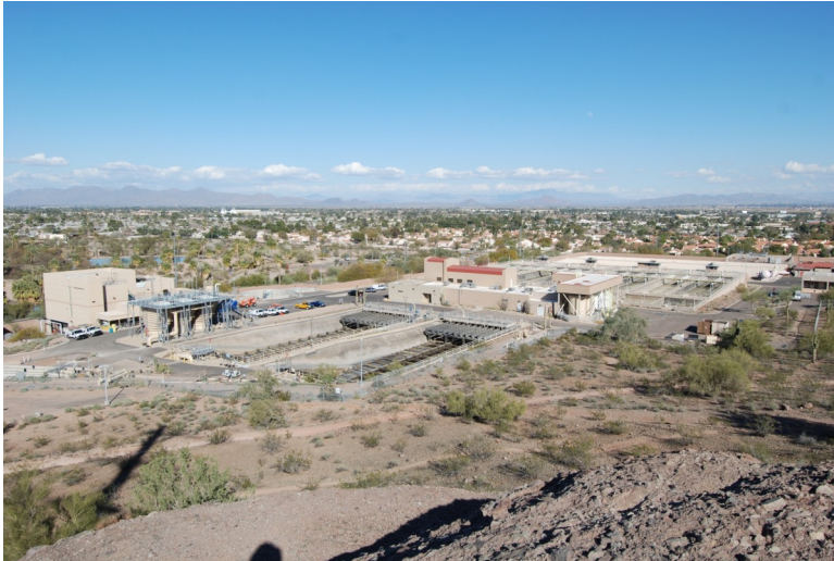
Tempe Johnny G. Martinez Water Treatment Plant
