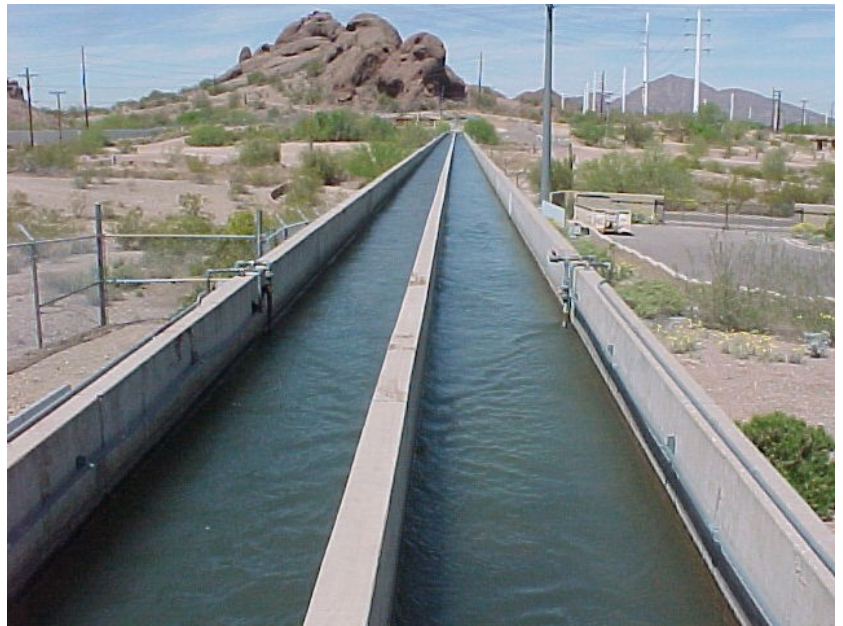
Flume from canal to Martinez WTP
