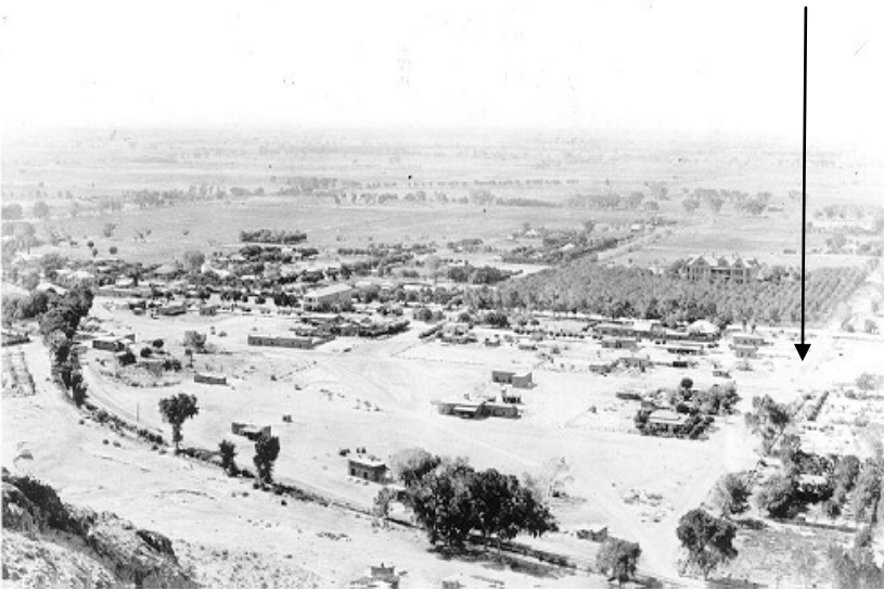
Tempe's first municipal well site (ca. 1902)
