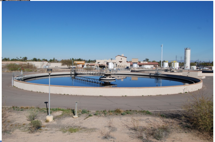
South Tempe Water Treatment Plant
